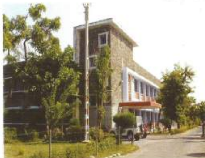
Basic Electrical School
