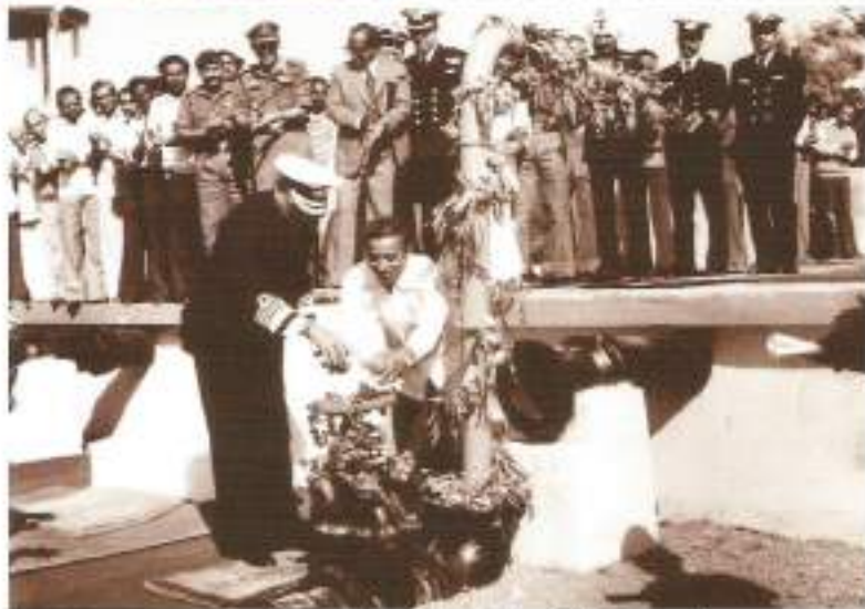
Inauguration of Sump by Admiral RL Pereira
