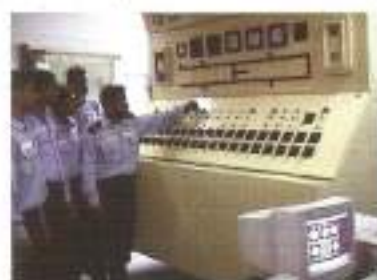
Training on Switchboard Simulator – Delhi Class
