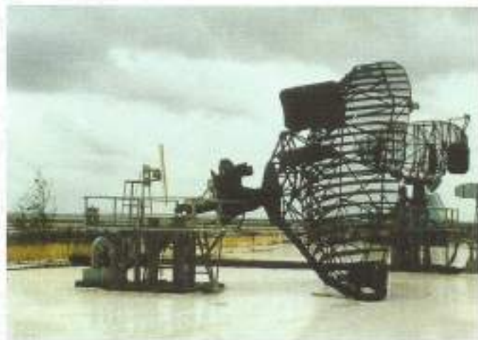
Radar Antenna Damaged After Cyclone
