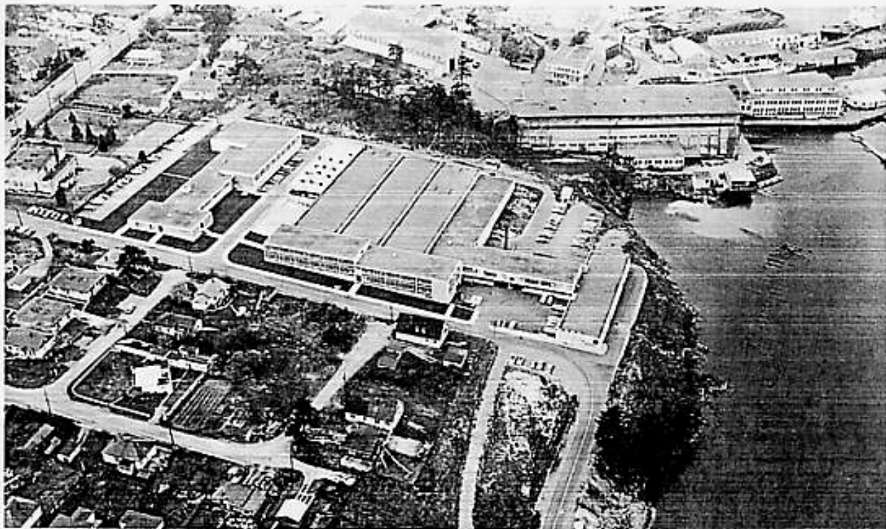
The Engineering Division of the Fleet School at Naden is located at the head of Esquimalt Harbour, not far from Yarrow's shipyard. (E-60695)
